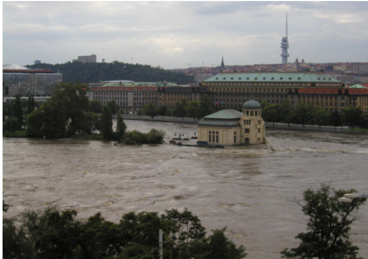
Historic Powerstation in Prague, flooded during 2002 Vltava flood. (Photo: V. Herle)
